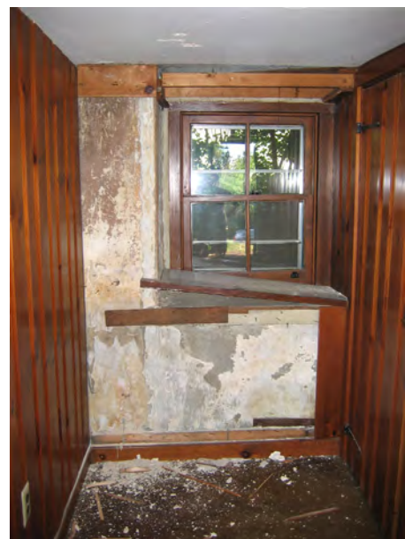
(RIGHT) Plate 6: Former exterior doorway.
