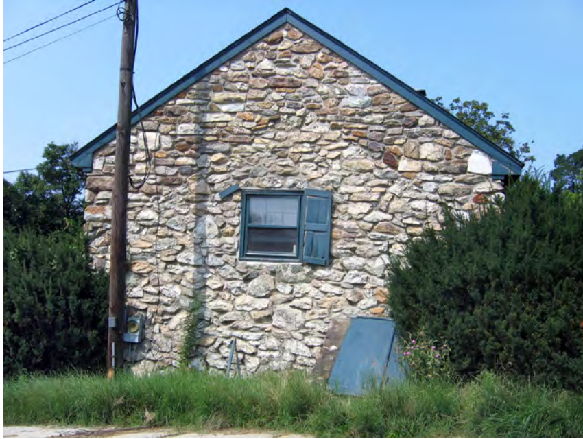
Plate 8: Former milkhouse, southeastern façade.
