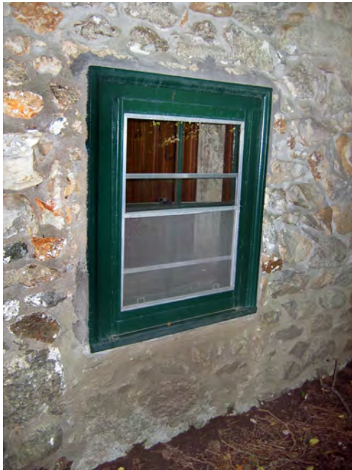
Plate 1: Converted window opening.
