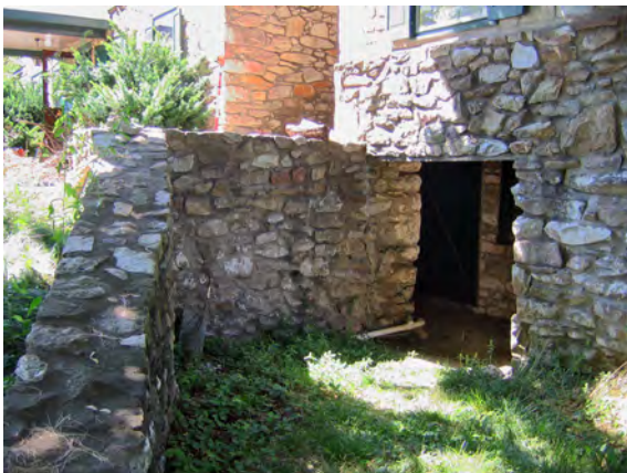
Plate 3: Exterior cellar access.
