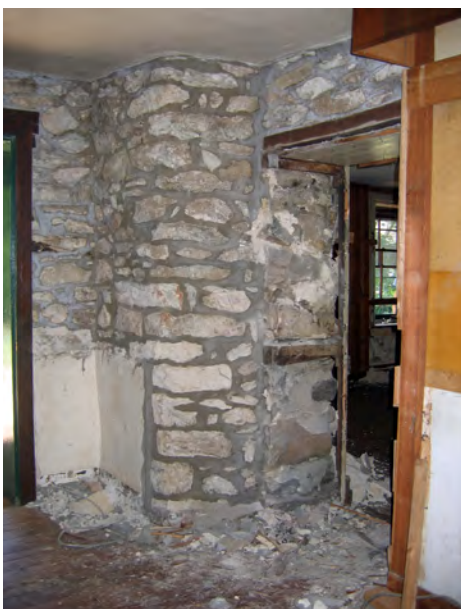
(LEFT) Plate 4: East wall of circa-1813 addition.
