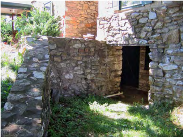
Plate 3: Exterior cellar access.
