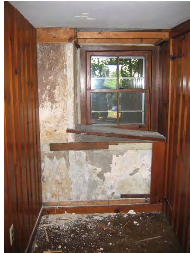
Plate 6: Former exterior doorway.
