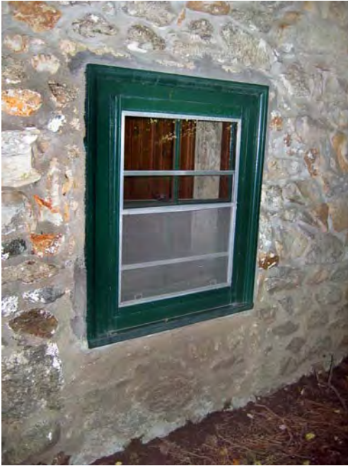
Plate 1: Converted window opening.
