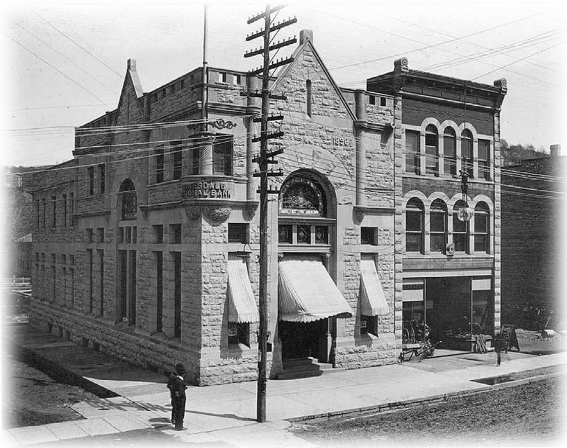
The Honesdale National Bank building, on the southeast corner of Main and Eighth Streets, was completed in 1896. The structure exhibits a mix of rough-faced and smooth stonework characteristic of the Richardsonian Romanesque style.
