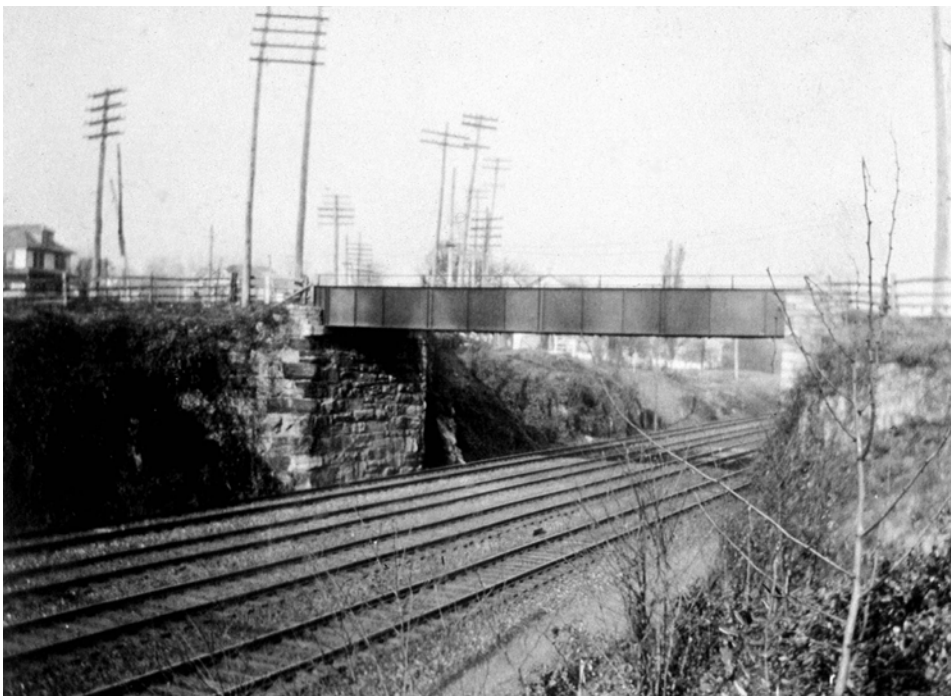
This is a northwestward view of the bridge that carried Lancaster Pike over the railroad tracks in Leaman Place from 1896 until 1923. To make it as short as possible, its builders placed the span on a 45-degree angle to Lancaster Pike, requiring travelers along the Pike to make awkward turns at both ends of the bridge. The structure blocks most of the Foundation Site house from from view.
