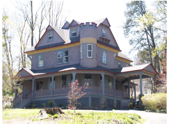
Note the shade provided by the porches and the surrounding trees. These elements keep the house cooler in the summer months.
